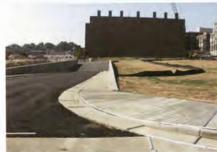
The Road to Somewhere Even before the Baptist rubble has been cleared (a little visible to the left) landscaping has begun. This new road has split the property and the new Pharmacy Building is to go up on the grassy area to the right.
